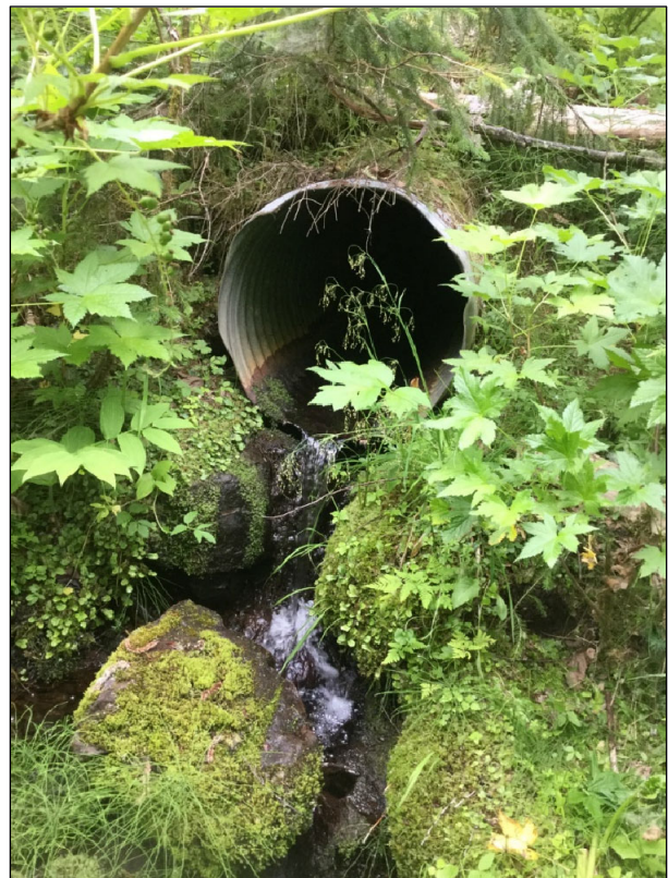
Figure 3.—Perched culvert outlet at waypoint 959.
